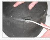
Put the cover on top of the fixture. Check for secure fit, and make sure the cover overhangs the hanger bars.
