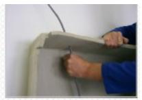
Place a single spacer, approx. 4"x4" (e.g. piece of ceiling tile, mineral wool batt) centrally located on top of the light fixture to provide a minimum 0.5" clearance between the light and the cover.
