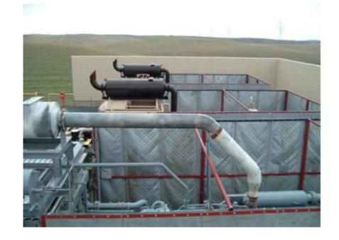
Typically used as modular sound curtain panels on long-term construction projects or permanent outdoor applications such as enclosing HVAC equipment, dust collectors or similar machinery where UV and abuse resistance as well as maximum durability, longevity and noise reduction is required. This product is also available with a one-inch thick quilted fiberglass absorber or with a two-pound per sq. ft. reinforced noise barrier.
