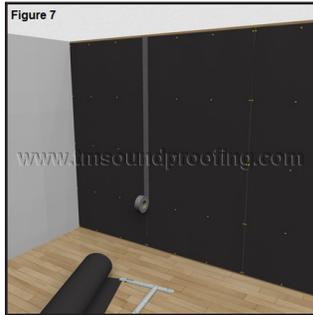
Where MLV seams fall on a stud, butt pieces against one another on the stud and fasten into place. You can add a strip of PVC Tape on the seam. {See Figures 6 and 7}
